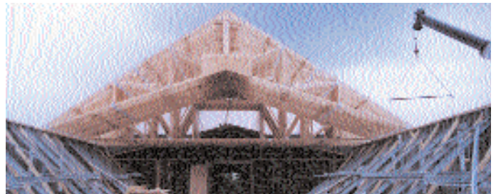
60' Scissor Trusses with plywood splice and braced walls
