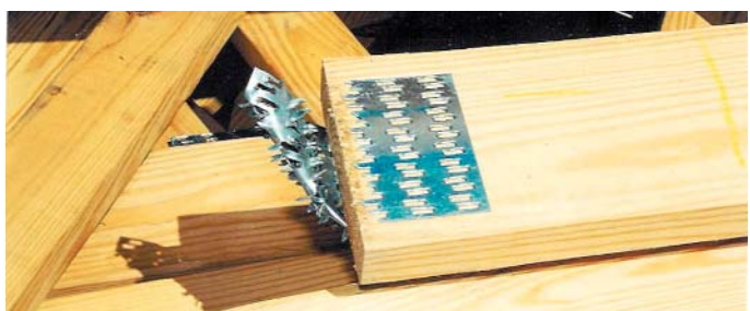
Broken BC Splice Plate
